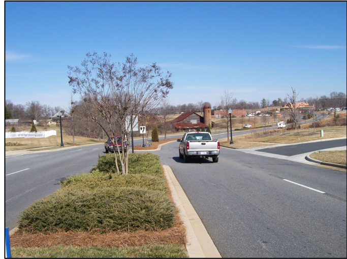
Morrison Plantation's four-laned residential roadway
