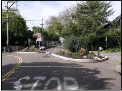
A traffic diverter on a Bike Boulevard in Berkeley, CA
