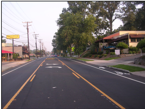
A lane conversion creates bike lanes and a new center turn lane from motor vehicle lanes.
