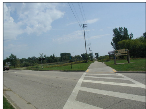
This rail trail intersection is more noticeable to motorists with this crosswalk
