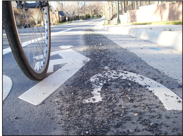
A system should be in place to sweep bike lanes and other bicycle routes and paths
