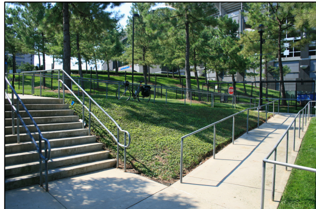
This wheelchair ramp at the Carolina Panther's stadium also benefits other users like bicyclists and parents with baby strollers.
