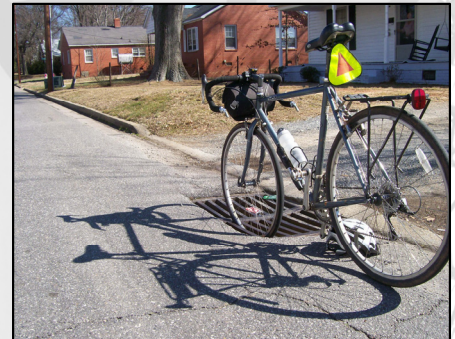
Roadways have hazards to bicycles.
