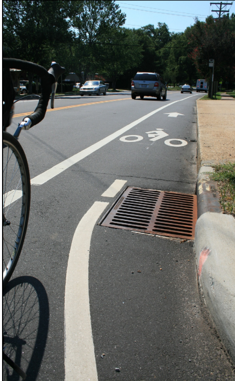
Dangerous grates, cracks, or holes should be fixed, while some hazards can be marked so that bicyclists can avoid them.
